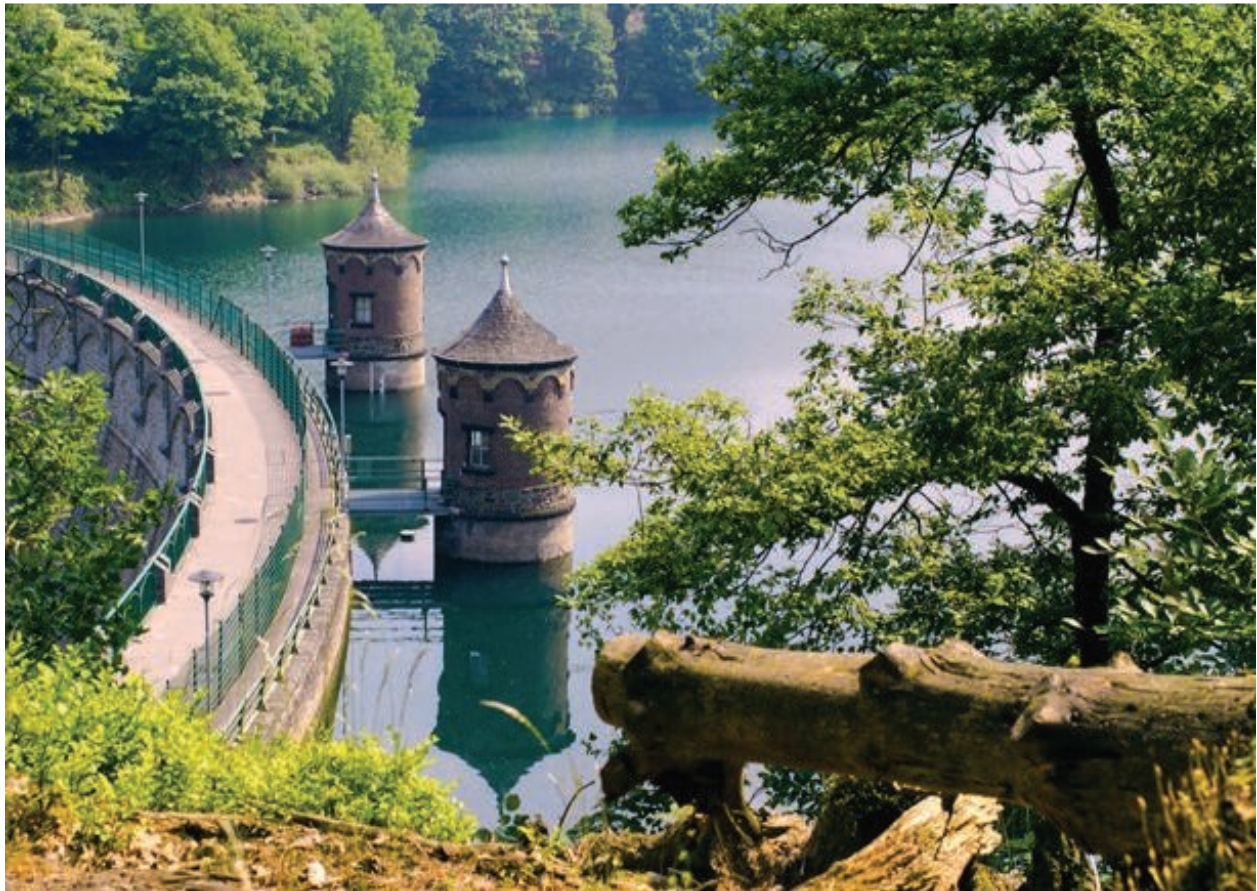
Sengbach Reservoir of the Glüder Waterworks
